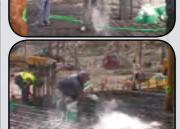
Apply MAXSEAL® SUPER by dry-shake method, providing a uniform coating on surface to be waterproofed.
